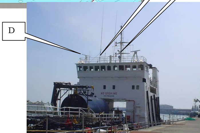
Figure 4.7: The Bunkering Tanker
