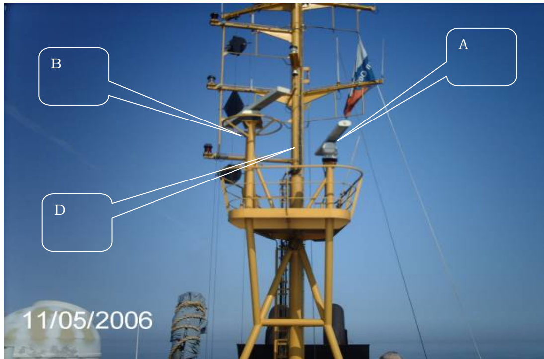
Figure 4.9: Dredger Antenna Installation
